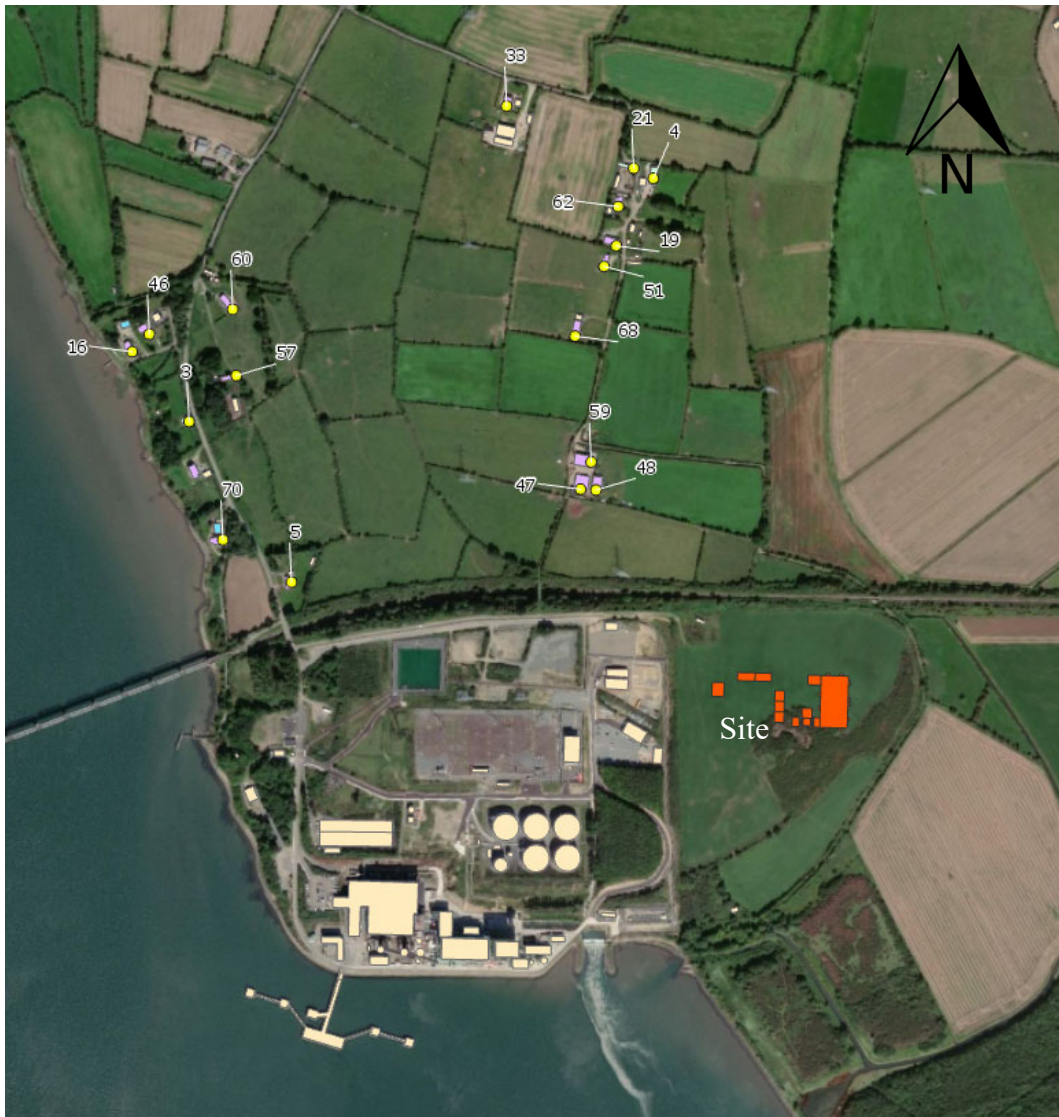
Figure 8.4: Receptors and Potential Receptors to the northwest of the Site | not to scale [mapping: Bing Maps © Microsoft 2020] (note that the nearest occupied residence is Receptor 68) (the worst-case configuration of the converter station was assessed and is indicated in this Figure)
